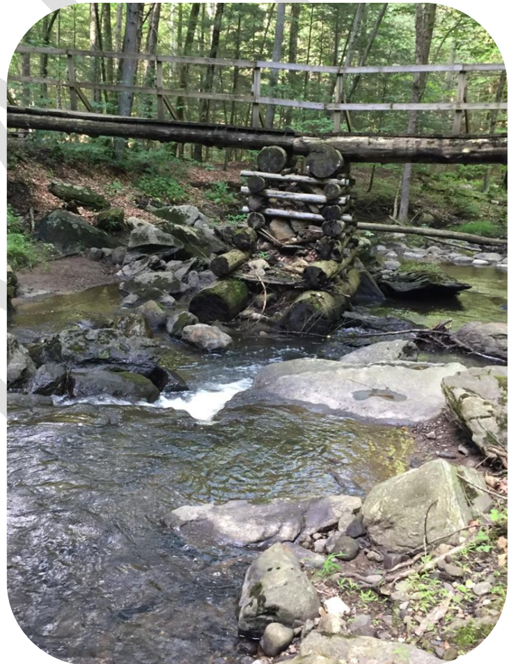
Appalachian Trail bridge over Deuel Hollow Brook.
