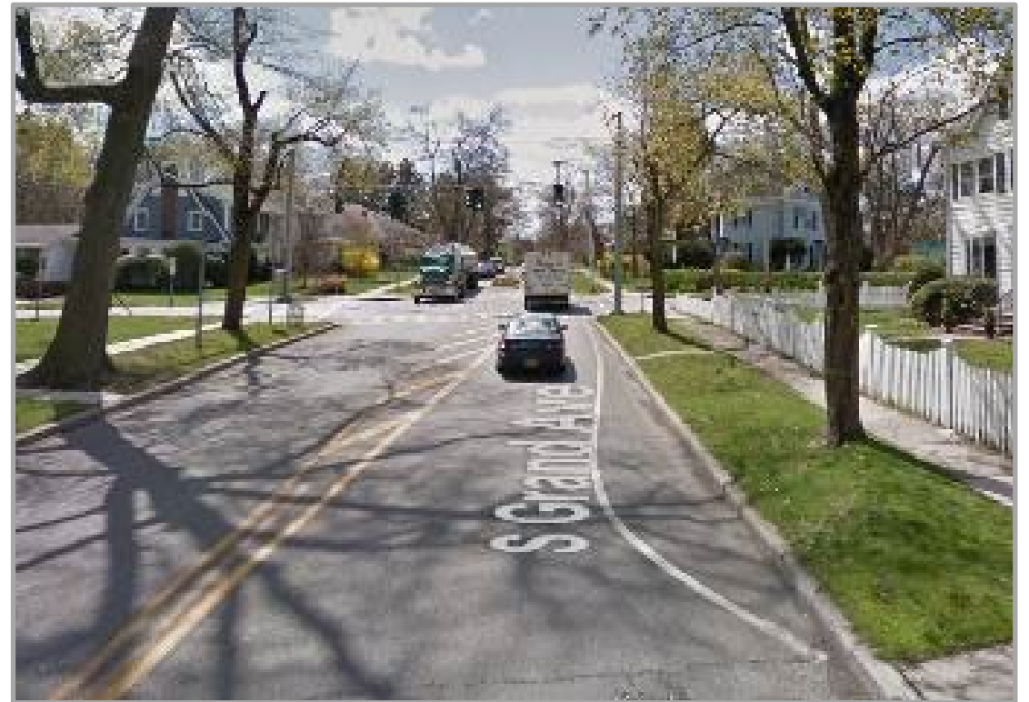
Simple pavement markings in the Town of Poughkeepsie help slow speeds (source: Google maps).
