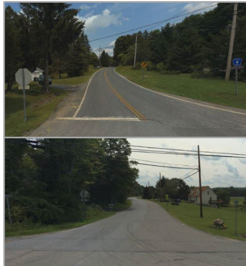
Lime Kiln Rd (lower photo) would benefit from striping, such as on Poplar Hill Rd (top photo).
