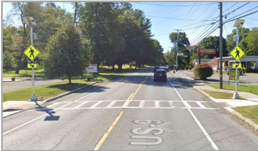
An example of Rectangular Rapid Flashing Beacons on Route 9 in Red Hook.
