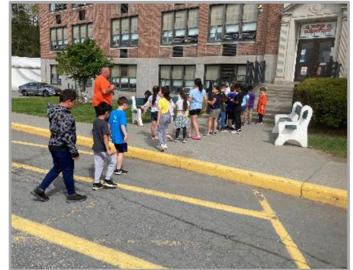
The Elementary School crosswalk lacks a curb ramp.
