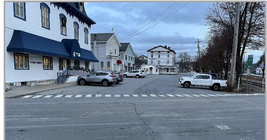
The newly marked crosswalk across Market St at Mill St would benefit from curb extensions to make people crossing more visible, given the adjacent parking.
