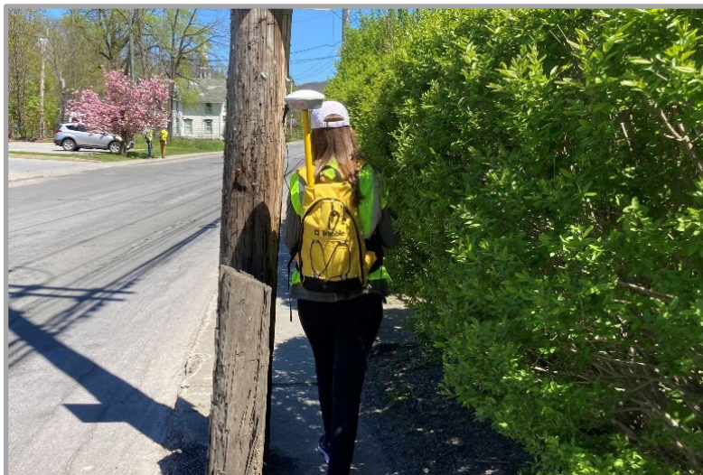
A utility pole and bush create an obstruction and limit clearance on the Mill St sidewalk near Route 22.
