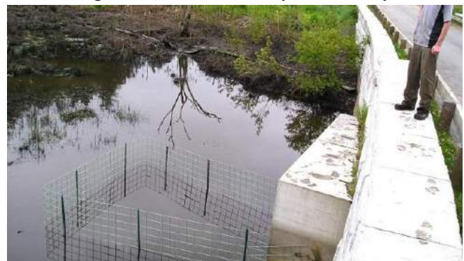
Culvert fences are the most commonly used beaver device by the Forest Service, however they may block fish passage. USFS concludes that the best solution is culvert replacement. Source: www.beaversolutions.com
